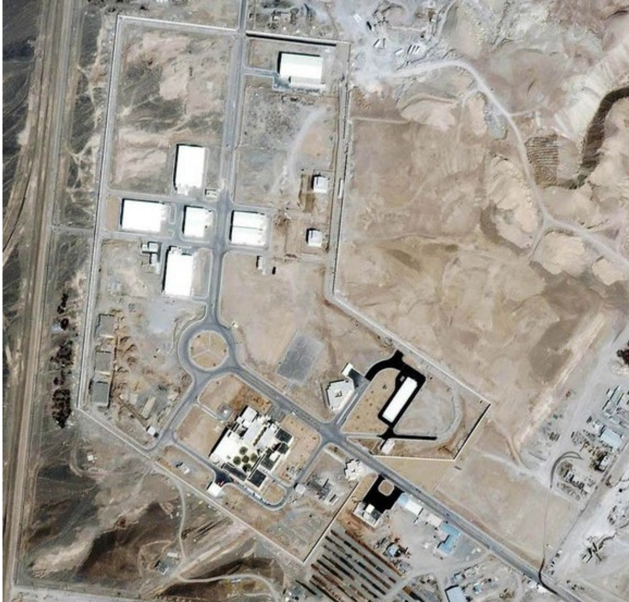
The once-secret nuclear complex in Natanz, Iran, about 150 miles south of Tehran
