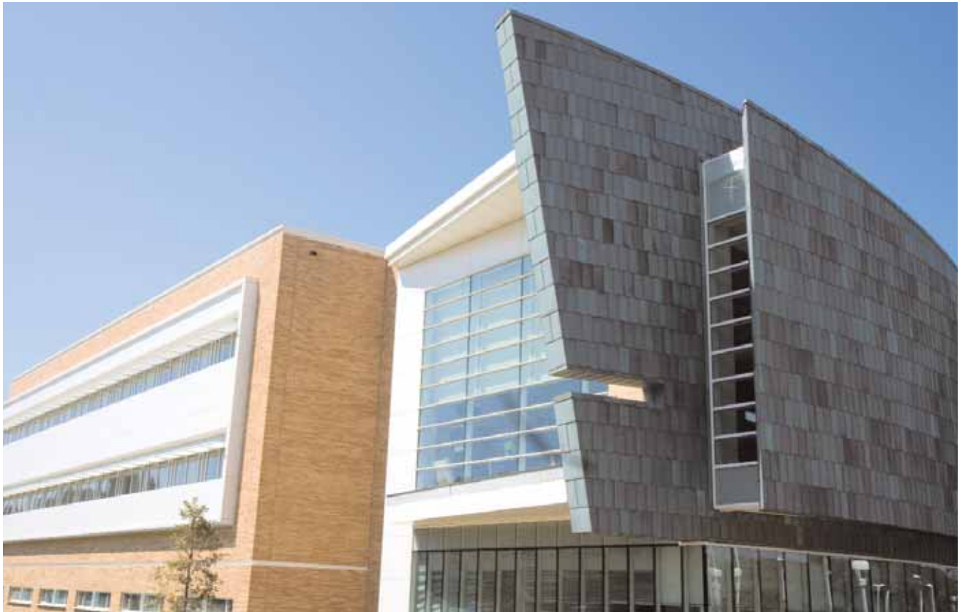
The Center for Excellence in Wireless and Information Technology (CEWIT) building.
